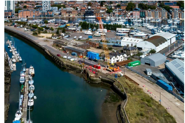
Quay Walls £16,300/m
